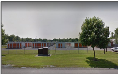
Cornwall Mini Storage Cornwall, ON 552 Units 42,528 SF
