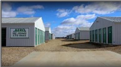
Aero Storage Camrose, AB 207 Units 30,680 SF
